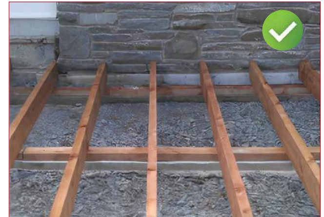
Bridging supports can be put in as required.
